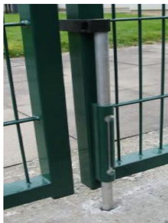
Picture 2: Ground bolt with housing
