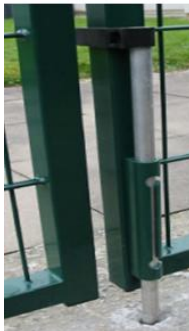
Picture 2: Ground bolt with housing
